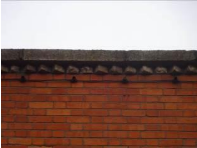
Fig. 9: Dogtooth course, north elevation
