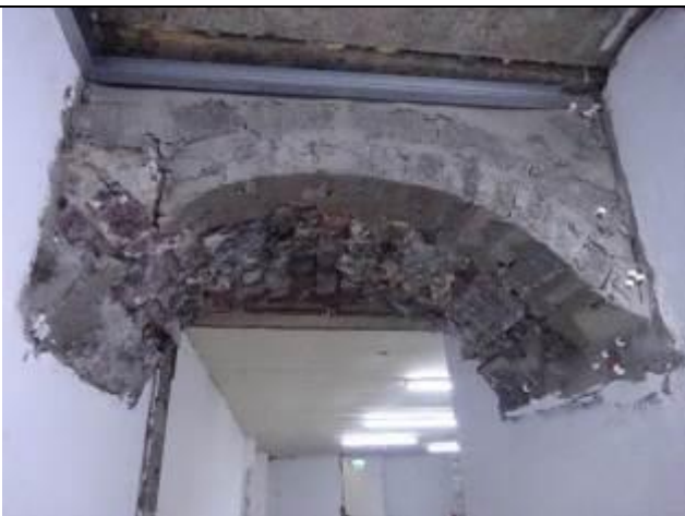
Fig. 19: Arch to opening in basement containing historic fabric
